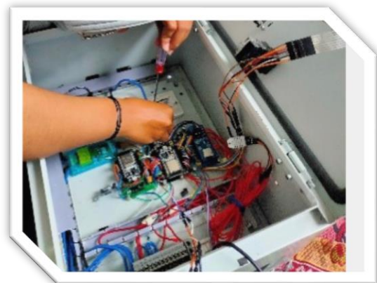
Gambar 2. Proses Instalasi panel
